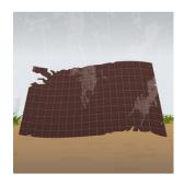
Inspect your plywood panels after each concrete pour and clean off any concrete residue. Avoid reusing severely damaged panels. Panels with light damage be can repurposed for making extensions.
